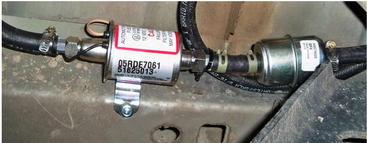
(Fig. 14) Fuel pump and inline filter installed.
