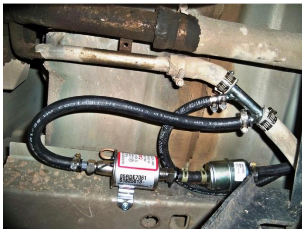
(Fig. 15) Vent Fill Neck Adapter installed.
