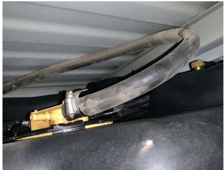
(Fig. 7) Lift tank high enough to reconnect electrical cable and vent hose to sending unit.
