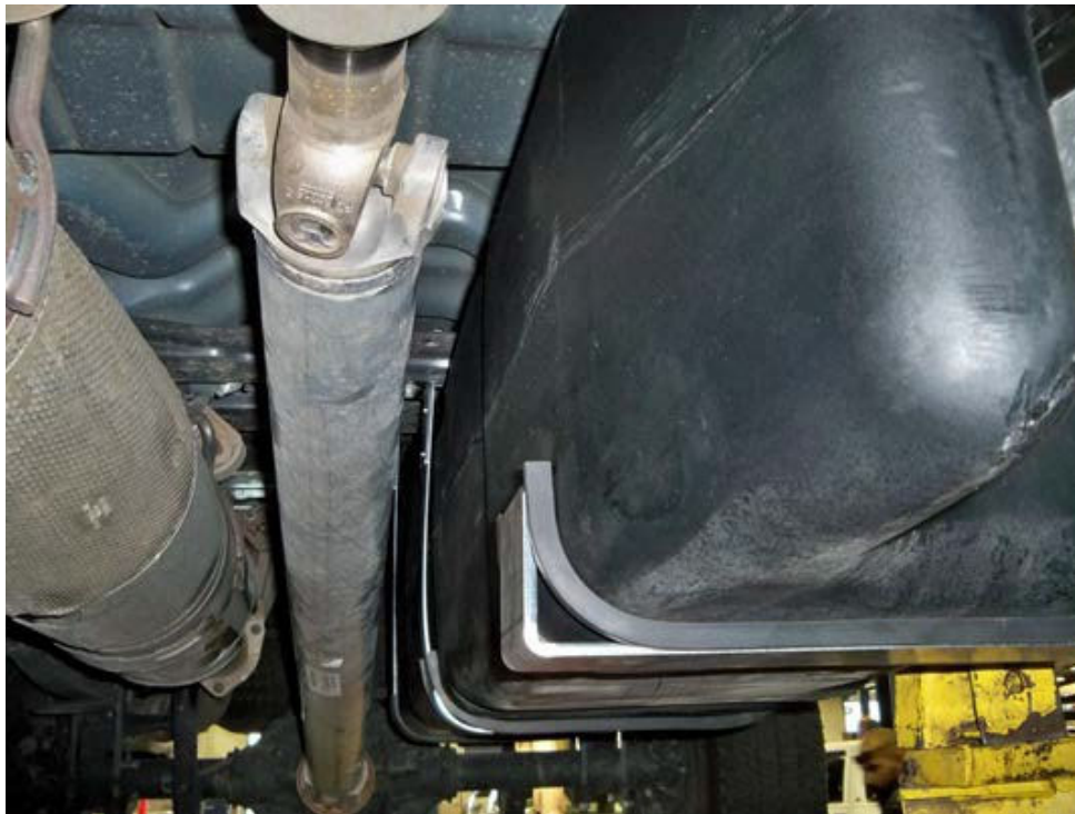
(Fig. 12) Installation of front support. Note the flexible bushings on the support and the straps.
